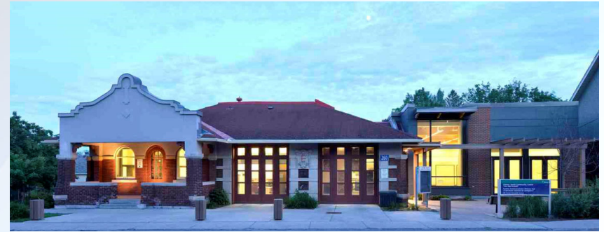
Old Ottawa South Community Centre
