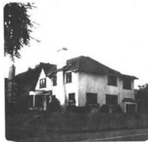
FIGURE 40 Island Park Drive Home (485 Island Park)
