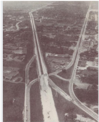
The Queensway in 1961 over Carling Avenue, following the completion of phase two
