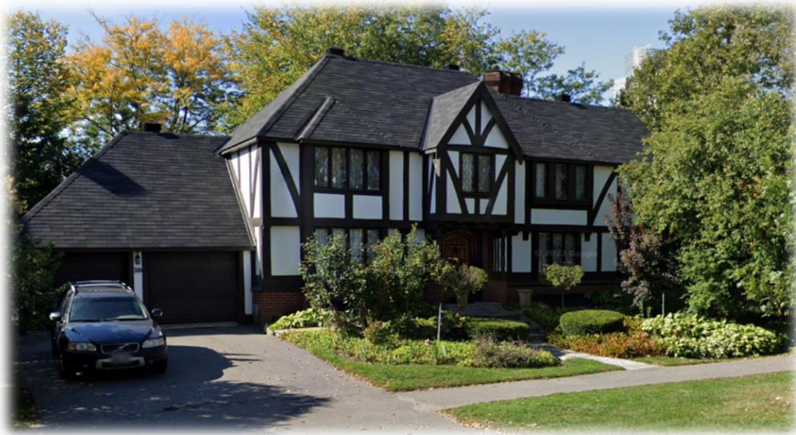
Tudor Revival 300 Island Park Drive
